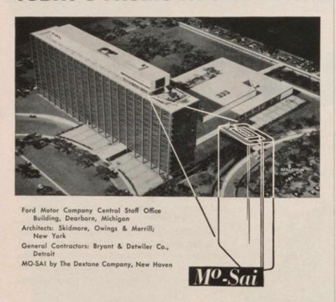
MO-SAI Precast Facing was literally wrapped around the structural columns of the penthouse of this striking new office building. MO-SAI's versatility of shape, size and color gives it an important place in today's architectural planning. MO-SAI Precast Facing combines the outstanding qualities of three dependable materials—Portland cement; granite or quartz aggregate; and steel rod mesh—in a factory-cast, rigidly controlled masonry slab with a remarkable versatility of application.
